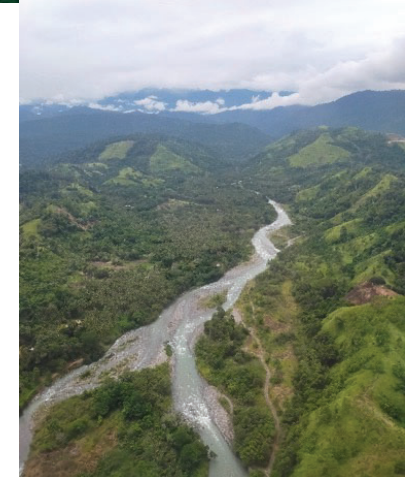
Kambara river for hydro power
